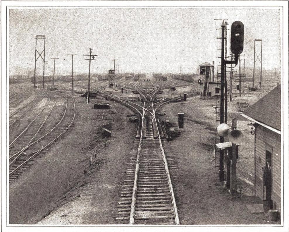
General View of Retarder-Equipped Hump at the Boston & Maine Yards in Mechanicsville, N. Y. Showing the Control Towers and the Classification Tracks
