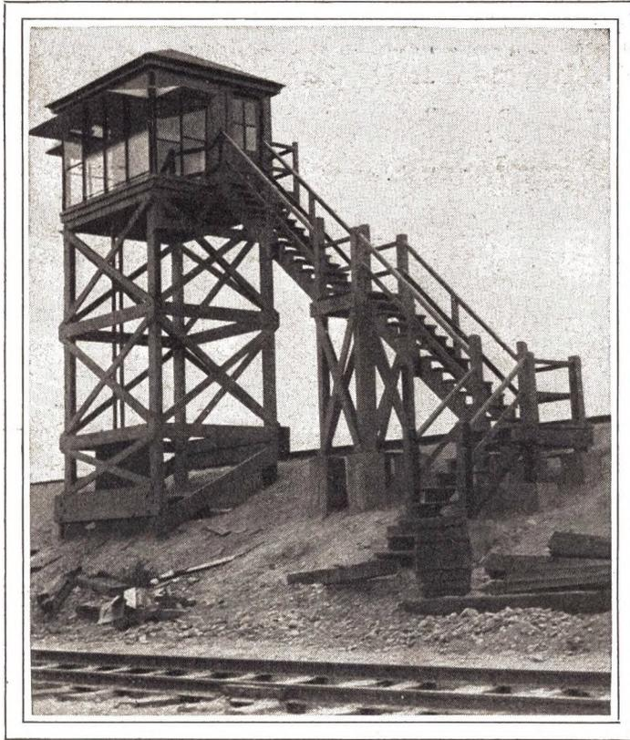
Typical Control Tower from Which Operations on the Classification Tracks Are Manipulated and Observed
